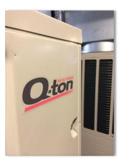
The installation was accomplished with a Q-ton unit along with a 2,000 litre tank supplied by MHI to meet the demand of 1,750 litre / day of the changing rooms and showers.
